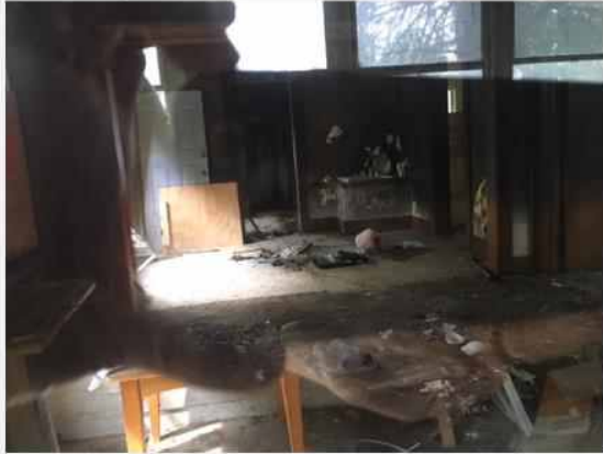
Inside the Living Room—through the front window
